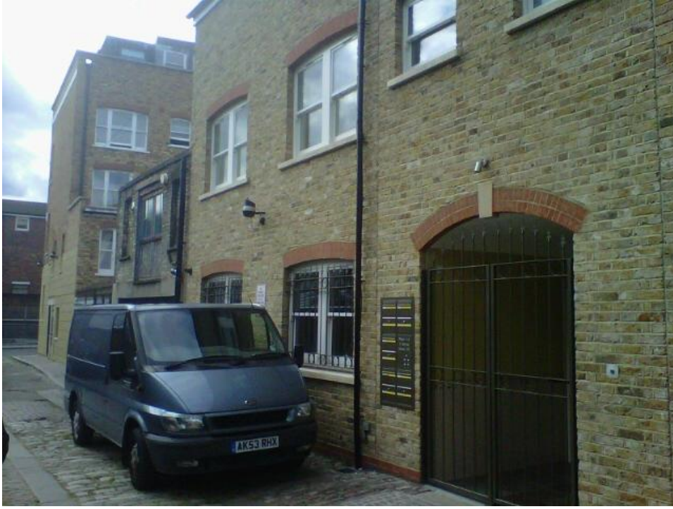
Image 4: Existing residential buildings at 1, 1a and 2 Moray Mews
