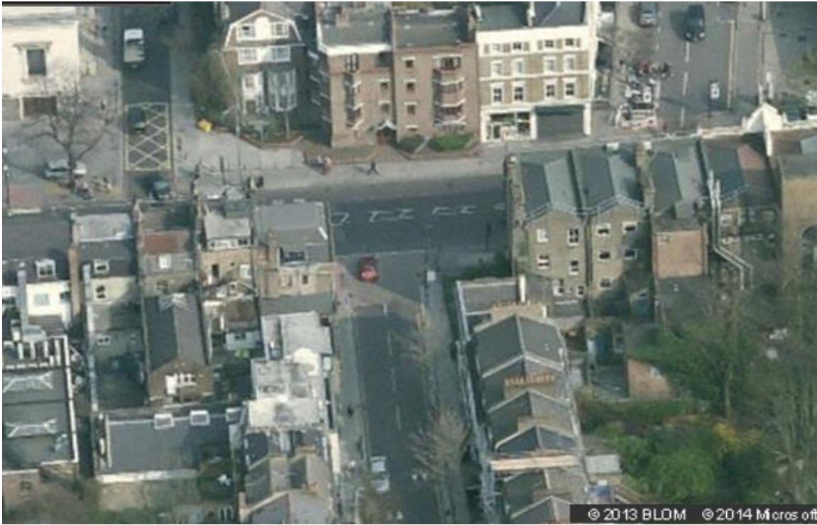
Image 3: View eastwards of existing application site.
