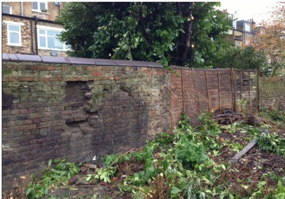
Image 5: Existing boundary wall / fencing to the rear of Moray Road
