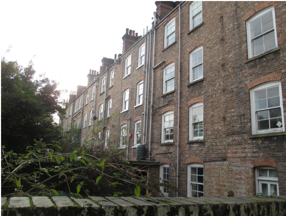
Image 3: Rear elevation of No. 17 and view to the south
